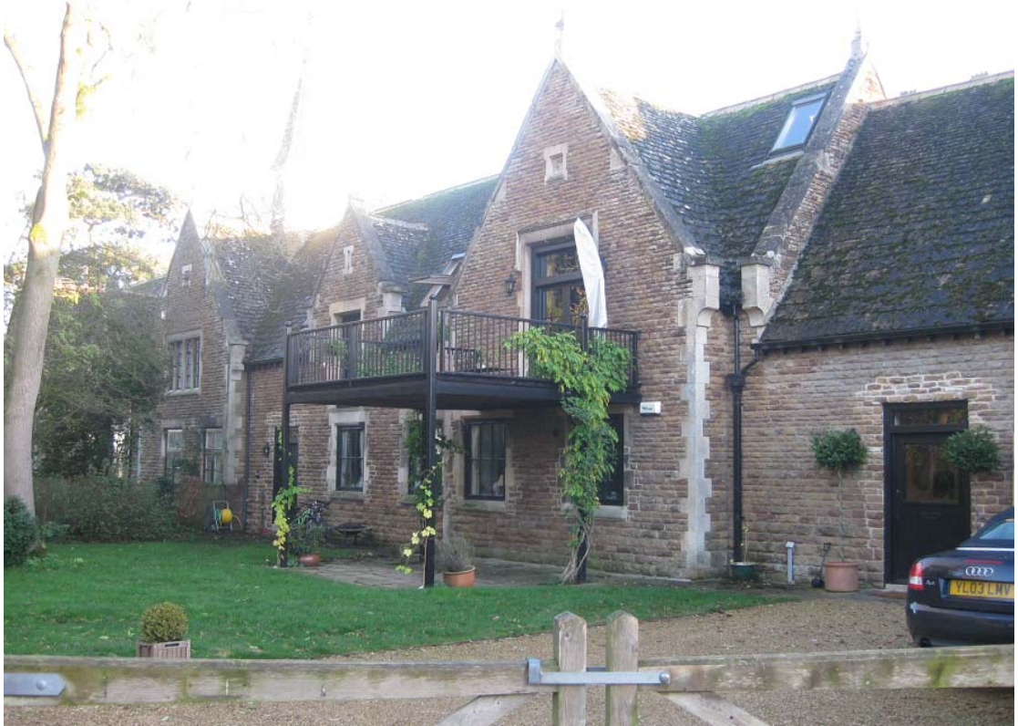
Current Unauthorised balcony
