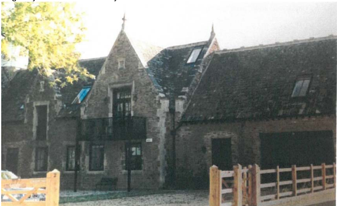
Originally constructed balcony
